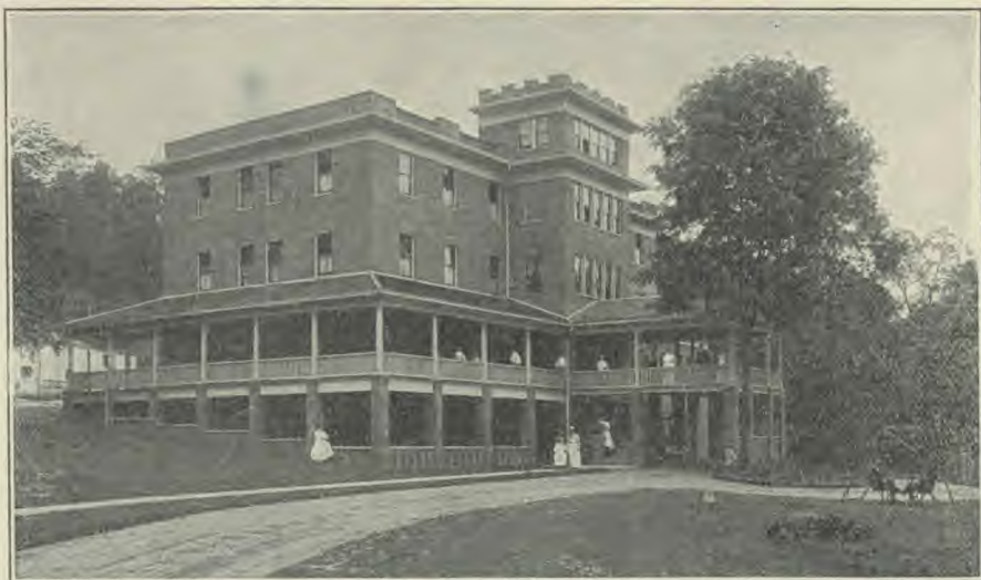
(One of Our Several Buildings)
