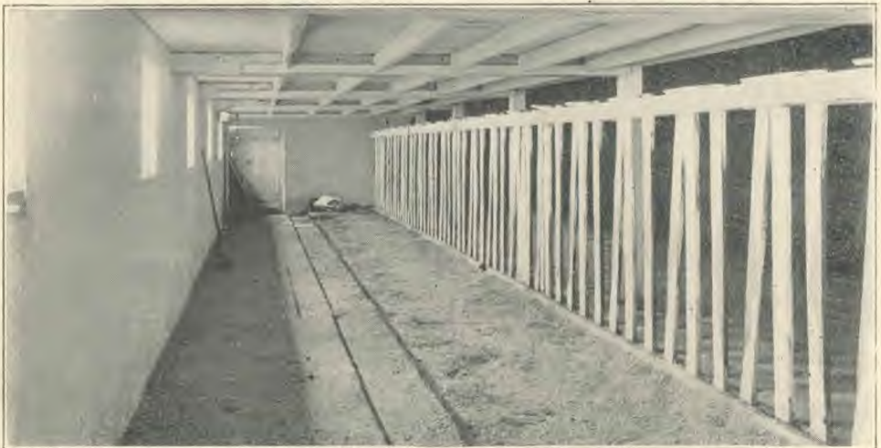
Stallway of one of the farms supplying committee's milk, just before cows enter. This room is kept sweet and clean, and produces milk normally under 50,000, usually under 25,000, and frequently under 500 bacteria per cubic centimeter. Room is whitewashed every two weeks, or oftener if necessary. Shavings used for bedding. Trough for offal, with drop-doors carrying offal to the tanks below. This keeps underpart of barn sweet and clean, and saves the manure for fertilizer, and prevents the breeding of flies
