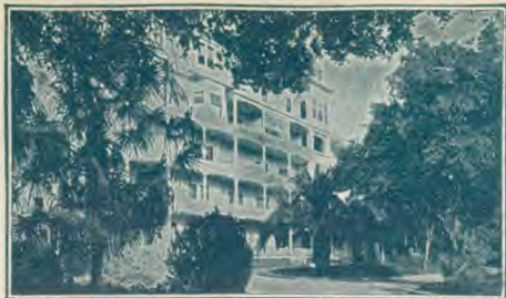
Part of Main Building
