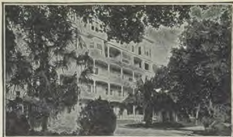
Part of Main Building
