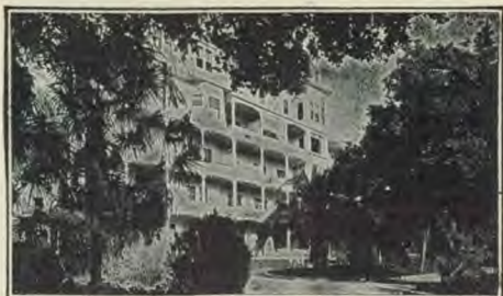
Part of Main Building
