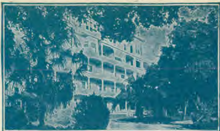
Part of Main Building
