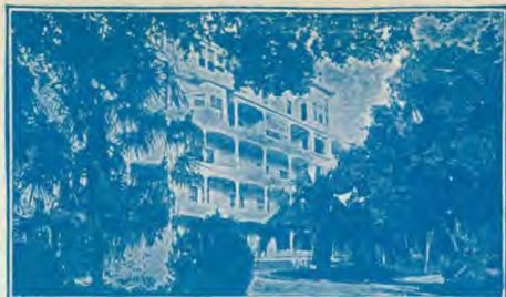
Part of Main Building
