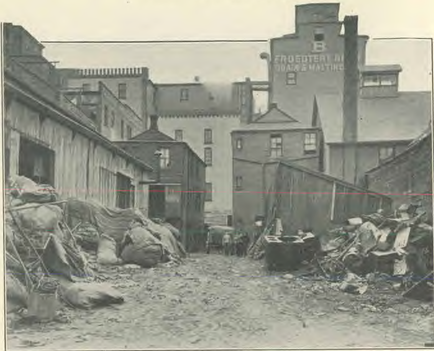
Rag-shop; barns, containing six horses; basements having dark rooms; water-closets in cellar, no light, no ventilation.
