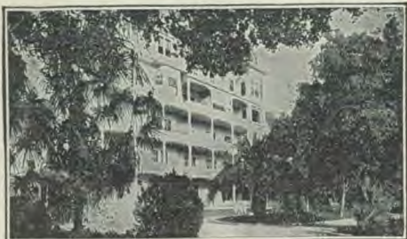
Part of Main Building
