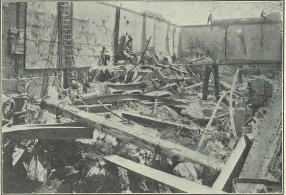
Unprotected steel in a supposedly fire-proof building.
