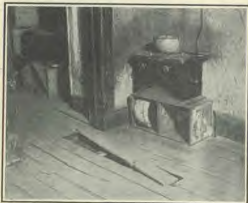
A poor man's kitchen — no light, no ventilation.
