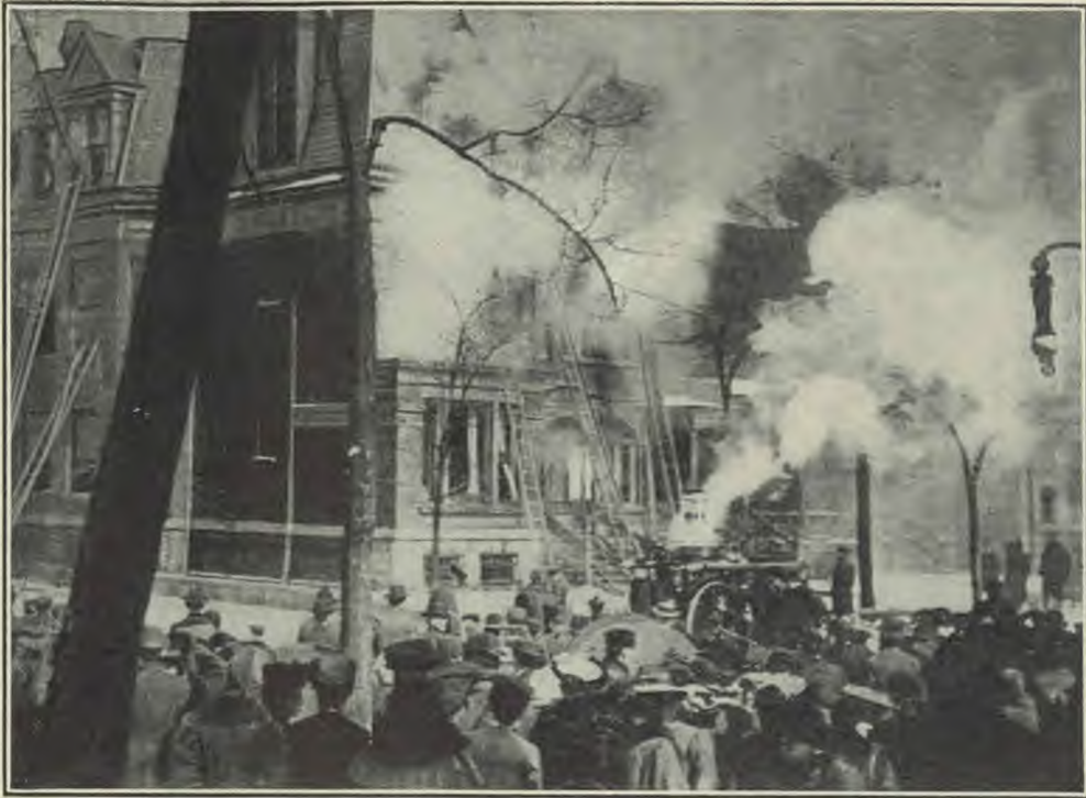
Hundreds of houses are burned every day because of faulty construction.
