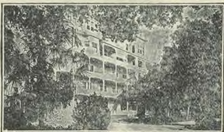
Part of Main Building
