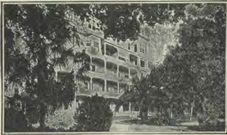
Part of Main Building
