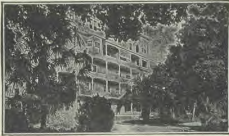
Part of Main Building
