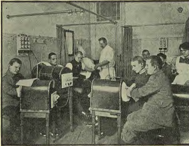
Apparatus for Applying Electric Hot-air for Stiff Joints
