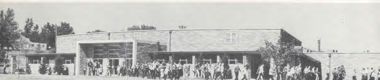
No place is more popular on Boys Ranch than the dining room. For uniformity's sake all buildings on the ranch are now being matched in architecture and materials used.
