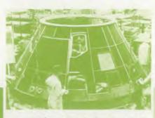
To keep it cool, the heat shield for an Apollo spacecraft is here assembled from fiberglass honeycomb panels of varying thickness, each injected full of a plastic ablative material to "boil' away damaging heat into space. Without the shield, astronauts would be exposed to temperatures as high as 5,000° F.
