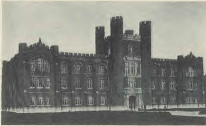
UNIVERSITY OF OKLAHOMA (NEW ADMINISTRATION BUILDING), FOUNDED 1892, REV. A. G. EVANS, PRESIDENT
