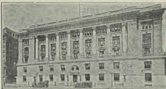
Post Office and Federal Building, Los Angeles, Cal.
