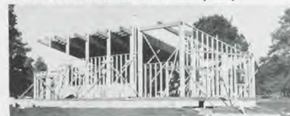
Pagosa Springs Church building under construction.
