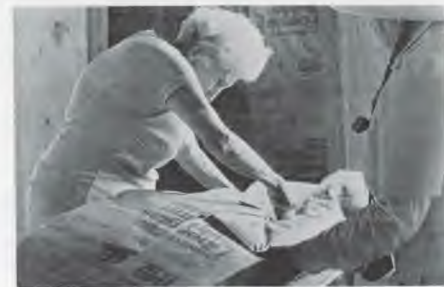
Insulation is measured and cut for the interior, and brickwork progresses on the exterior.
