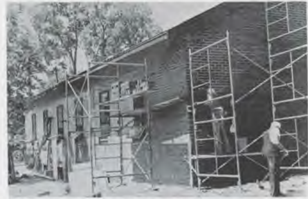
Insulation is measured and cut for the interior, and brickwork progresses on the exterior.
