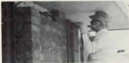
Ernie Seltmann laying bricks.
