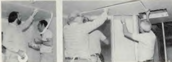
Lee Thompson, Dwight Mayberry, Jean Avey and Joel Tompkins install sheetrock.
