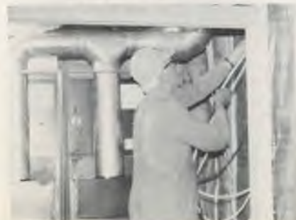
Willis Mohr pulling electrical wires.
