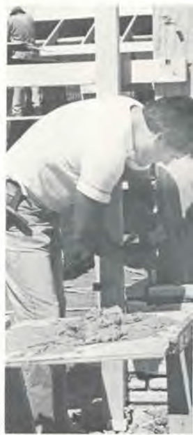
Frank Martinez, dean of boys at Enterprise Academy, worked at laying brick.
