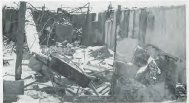
All that remains—ashes, twisted pipes and concrete walls—of the Watford City church.
