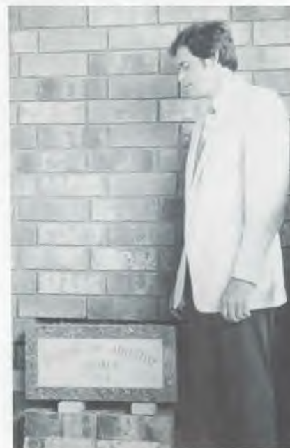
LeRoy Wood, contractor, standing by the cornerstone.
