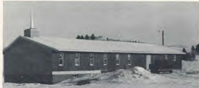
Pine Ridge Mission church nearing completion.
