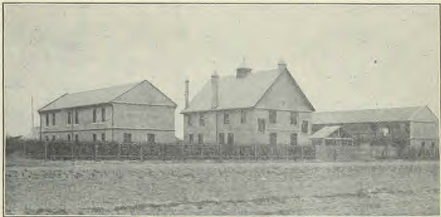
THE SCHOOL BUILDINGS NEARING COMPLETION
