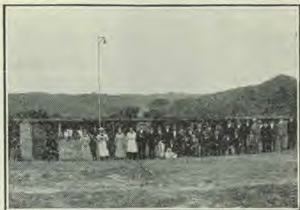
THE CHICKEN HOUSE, TEMPORARILY OCCUPIED BY THE WORKERS
