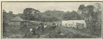
BEGINNING WORK ON THE SCHOOL FARM
