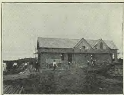
WORKING ON THE SCHOOL BUILDING
