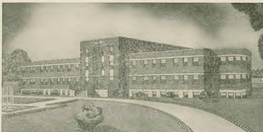
The New Riverside Sanitarium and Hospital Now Being Constructed
