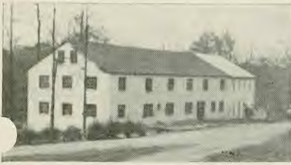
New Boys' Dormitory Under Construction, Pine Forge Institute
