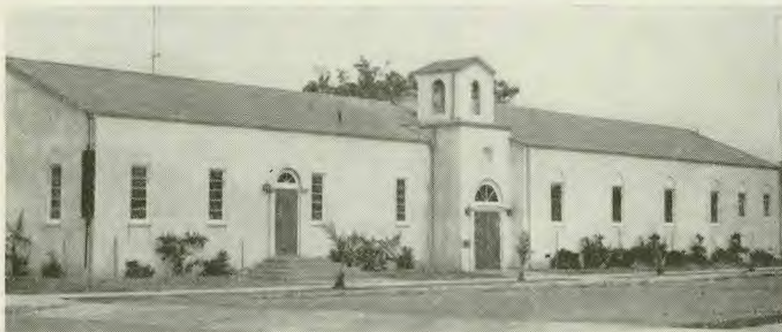
Nearly all the members helped and sacrificed personally to erect the church in San Bernadino.
