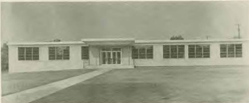
PHOTO BY PINKNEY New Cleveland intermediate school on Lee Road near Miles. Estimated value, $160,000.
