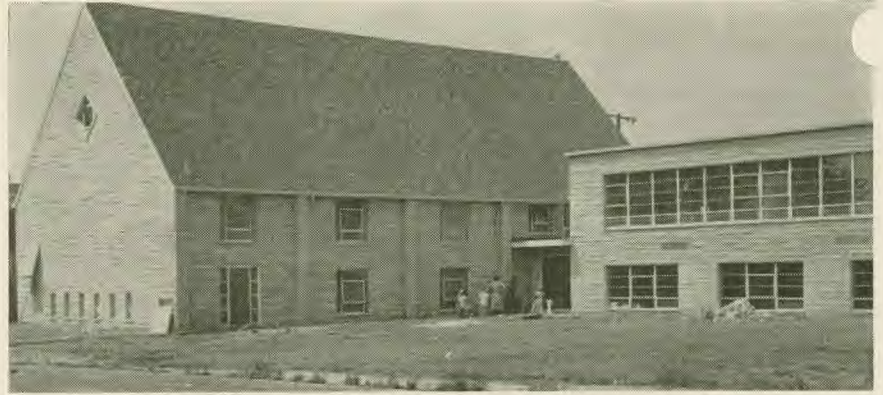
Mizpah church and school building under construction in Gary, Indiana.
