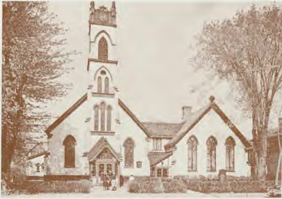
Rochester church is landmark of city, easily accessible by public transportation. Property was purchased for $65,000.
