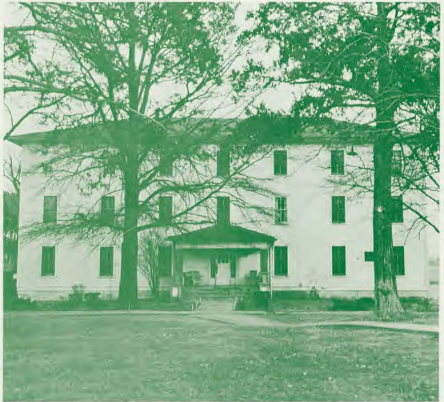
Henderson Hall now condemned.
