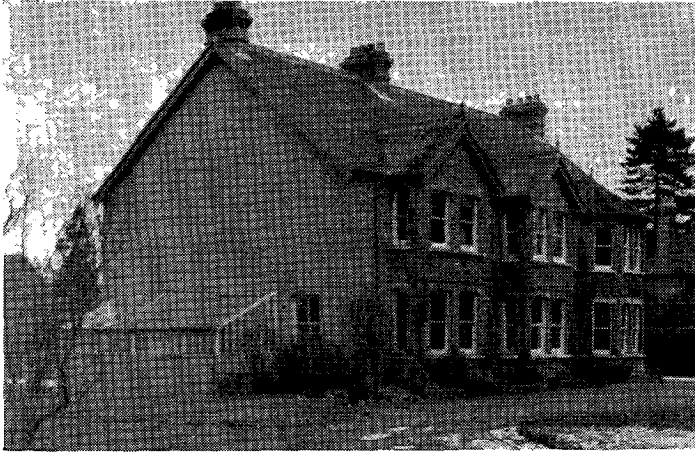
"Crossways" — a new residence housing, at present, six married couples and their children.
