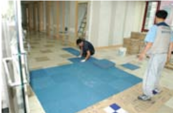
Fifth floor new office area getting carpet in preparation for occupancy
