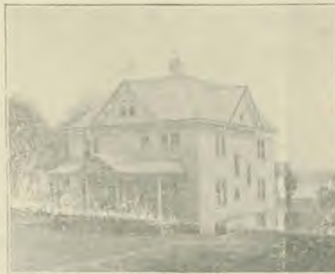
Main School Building, Mipewoak Academy
