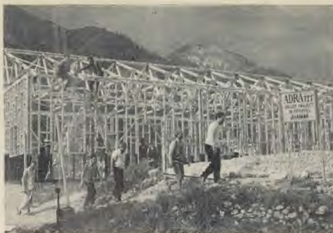
A community hall built for the earthquake victims at Uttarkashi.
