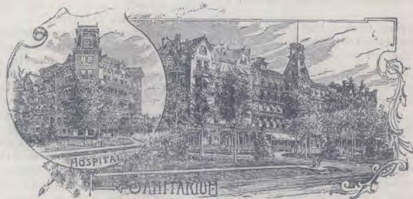
TWO MAIN BUILDINGS OF THE BATTLE CREEK SANITARIUM.
