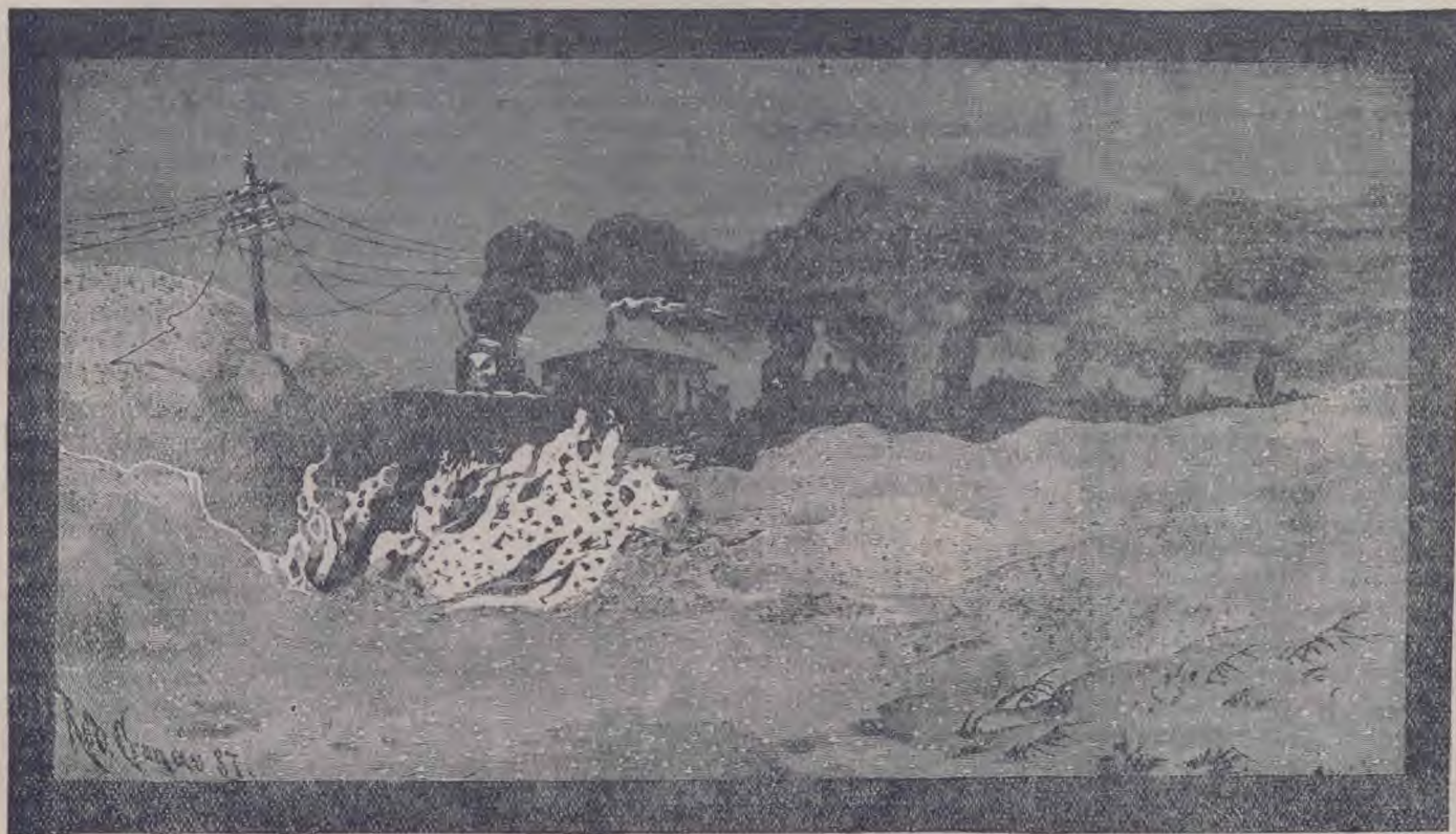
Locomotives with Snow-Ploughs clearing the Line.
