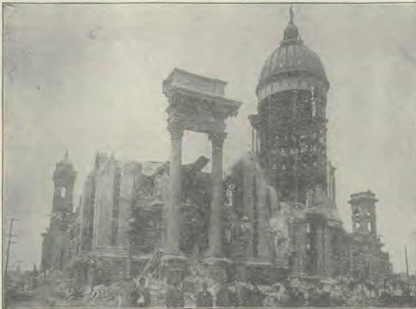
Result of the Earthquake, San Francisco
