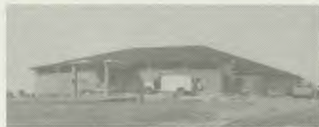
The completed structure of the New Heights SDA Church in Jackson, Mississippi.
