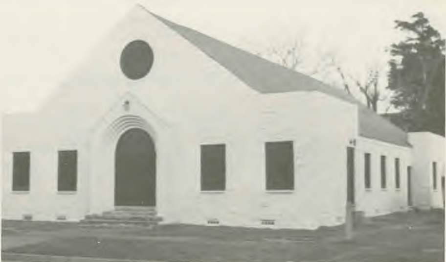
Berean (Houston) completely renovated and reopened.
