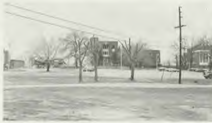
The old Riverside building was razed.
