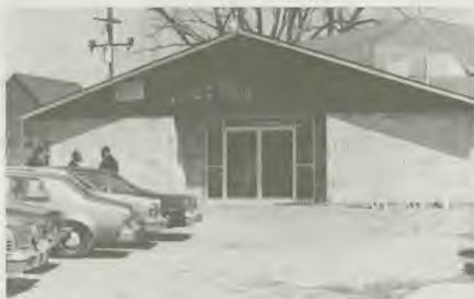
The Conant Gardens church in Detroit, Michigan, still under construction.
