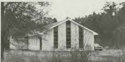
The newly constructed Memorial SDA Church in Mansfield, Louisiana.
