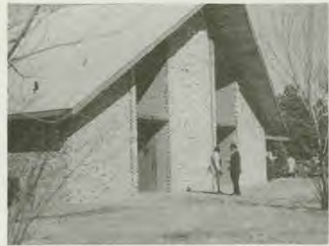
Church Buildings — From 1976-1985 31 churches completed and 22 more on the drawing board. (Pictured Tulsa, Oklahoma Church 1st church purchased in 1976.)
