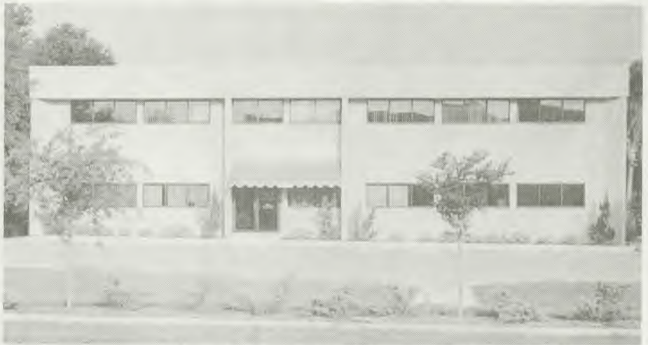
Home headquarters for Southeastern Conference, Altamonte Springs, Florida.
