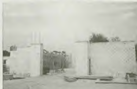
North Orlando SDA Church under construction. Opening scheduled for July, 1988.
