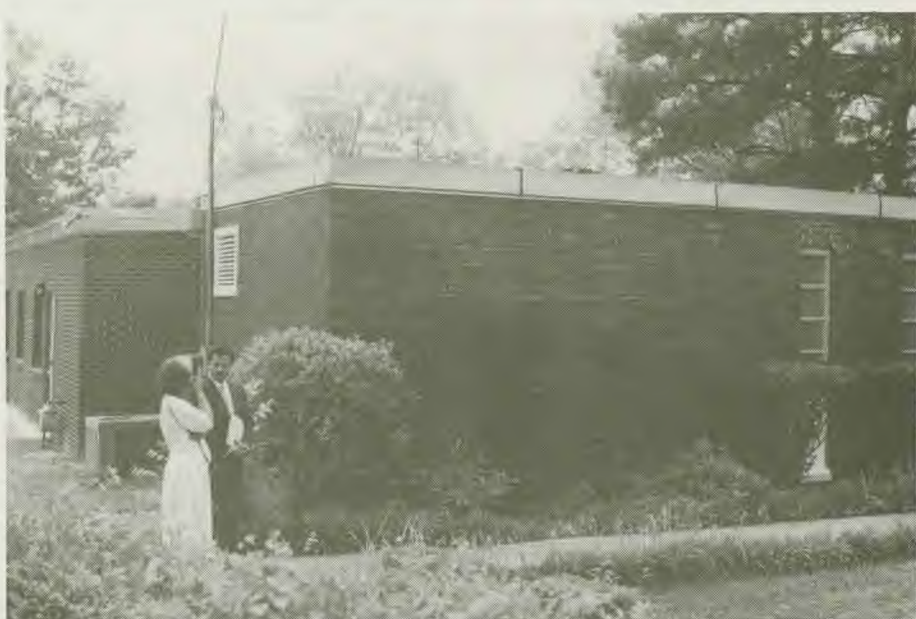
Maranatha building, Montgomery, Ala.
