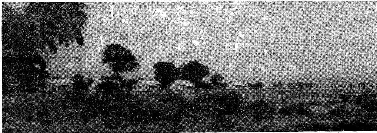
A view of the Raymond Memorial Training School, Falakata.
